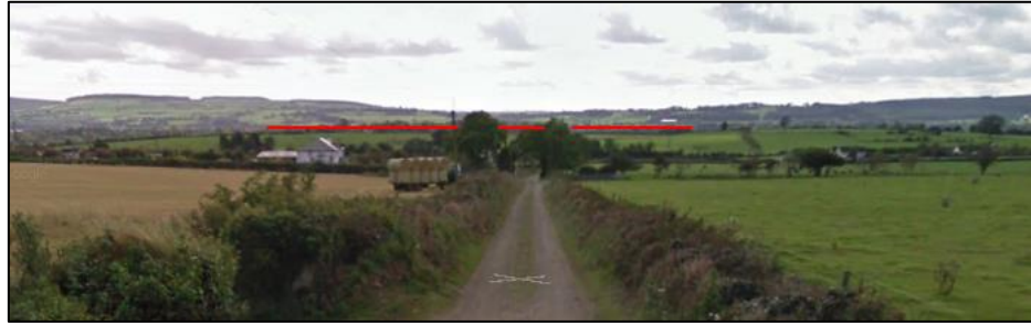
Figure 3: View to southern parcel from entrance to northern parcel (indicative site boundary in red)
